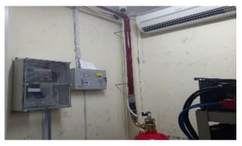
Figure 6: Newly installed FM 200 fire suppression system- Switch room
