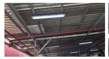
**Figure 4:** Fire foam sprinkler system installed at the finished goods warehouses
