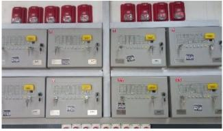
*Figure 3:* Generator House- Newly installed Gas/Diesel Engine Auto DCP Fire Suppression system
