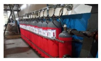
**Figure 2:** Newly installed Morpack W&H auto CO2 suppression
