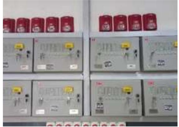
Figure 3.26: Generator house - newly installed gas/diesel engine Auto DCP fire suppression system
