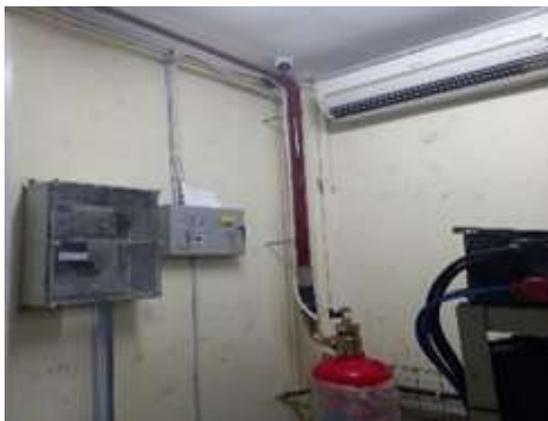
Figure 3.29: Newly installed FM 200 fire suppression system - switch room
