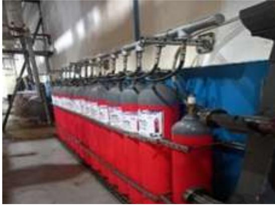
Figure 3.25: Newly installed Morpack W&H auto CO2 suppression
