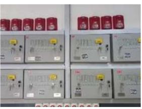
Figure 3.26: Generator house - newly installed gas/ diesel engine Auto DCP fire suppression system
