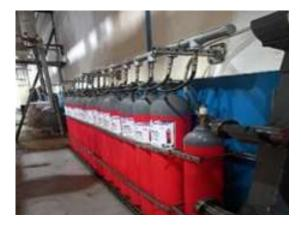
Figure 3.25: Newly installed Morpack W&H auto CO2 suppression
