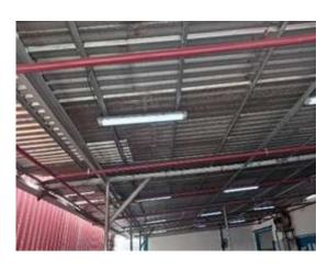
Figure 3.27: Fire foam sprinkler system installed at the finished goods warehouses
